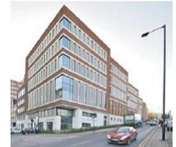
Graduate School (Sheffield University) Sheffield (United Kingdom) Architects: Brond Bryan Architects
