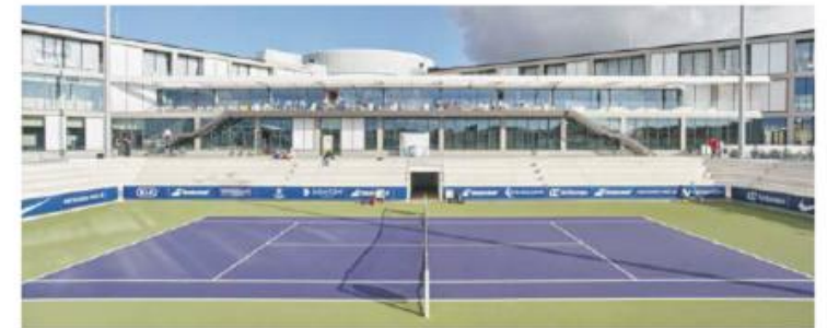
Sports Centre Rafa Nadal Manacor - Illes Balears (Spain) Architects: Bimbe / Talat (Engineering & Project Management)
