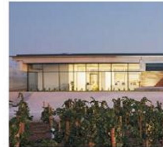
Beronia Rueda Winery Rueda - Valladolid (Spain) Architect: IDOM
